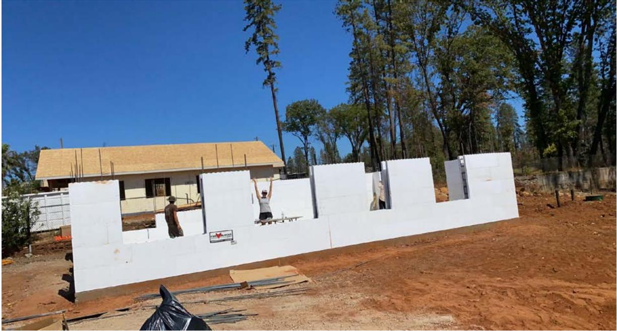
*Figure 8: Top of the ICF forms built and placed*
