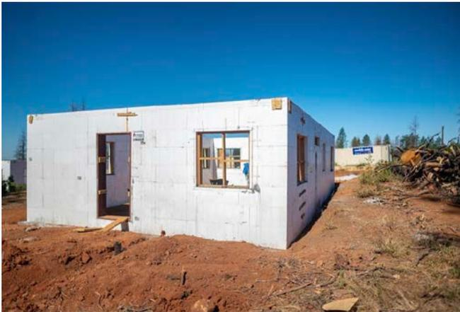
*Figure 1: Insulated Concrete Form Home*
