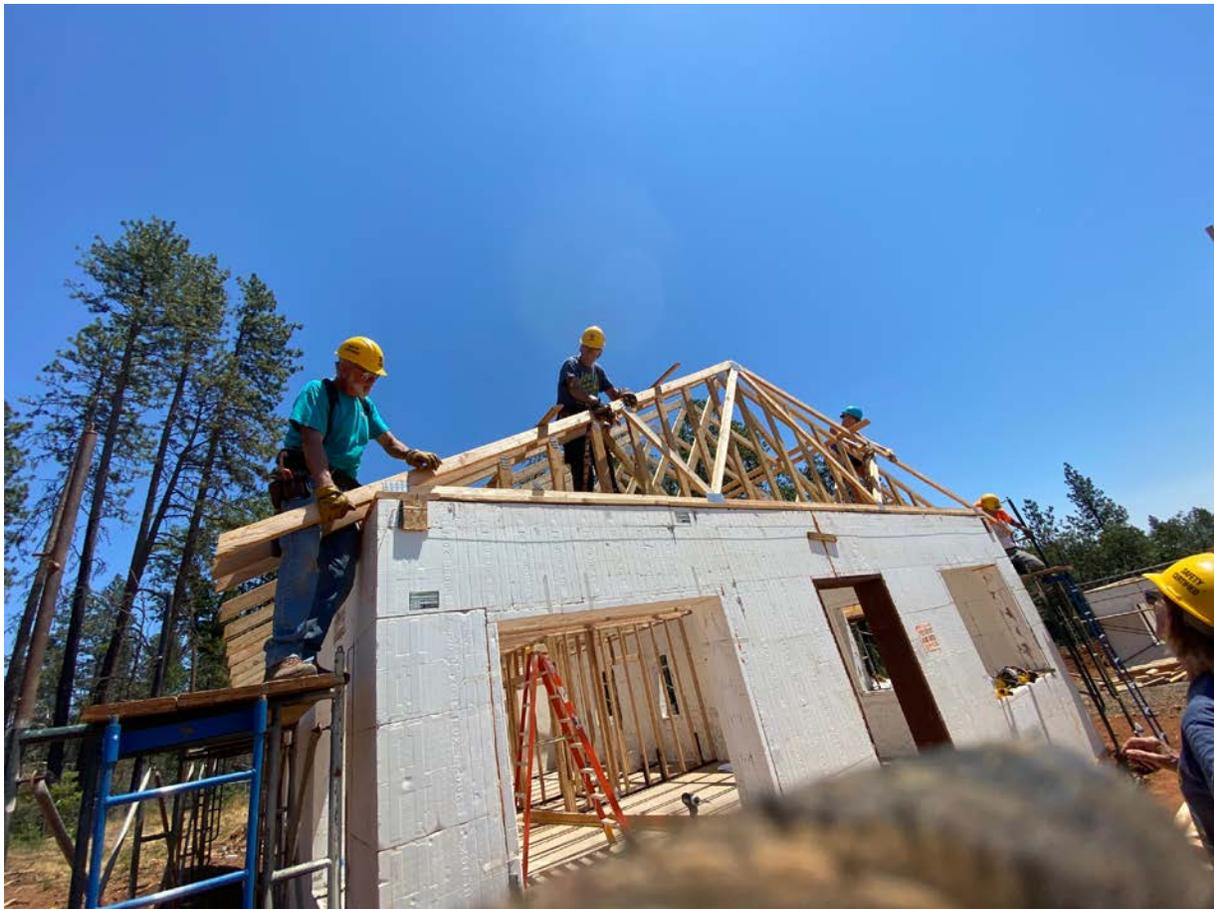
*Figure 5: Caravanners and I rolling trusses*
