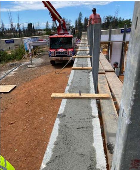
Figure 4: Inserting bolts and screeding excess concrete
