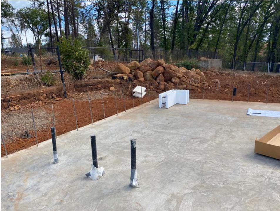
*Figure 6: Making lines for the ICF*
