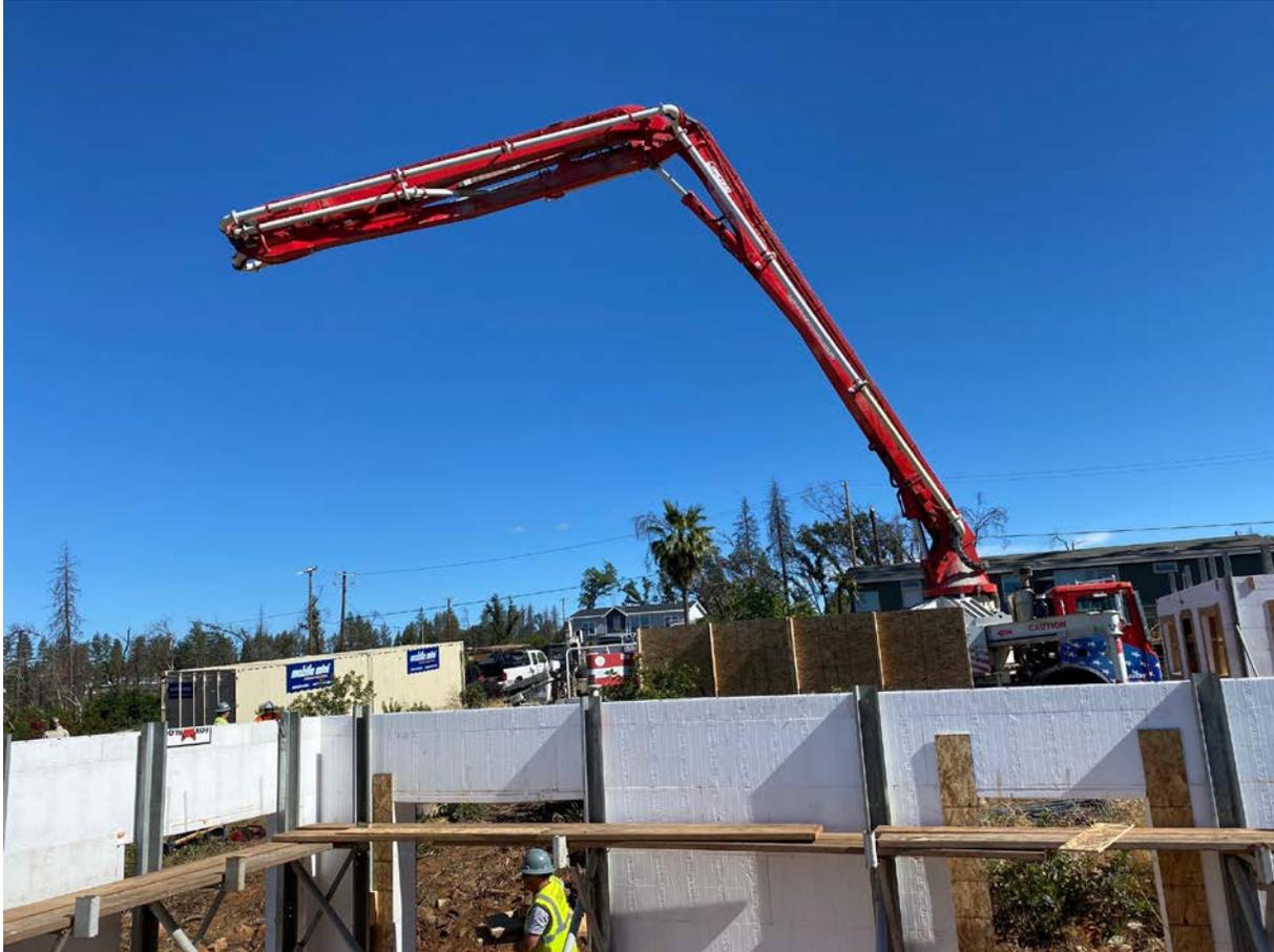
Figure 3: Pump concrete truck
